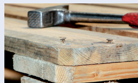
Hammering down projecting fastening elements
