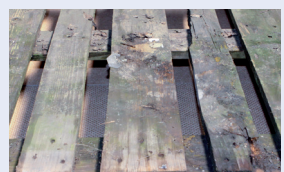
Drying/cleaning soaked boards
